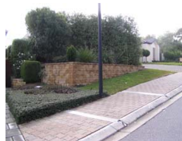
Minimise the height of retaining walls and use materials that blend with the natural environment
