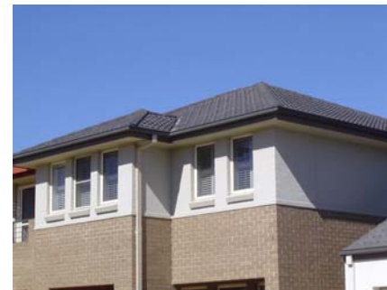
Eaves shade windows and assist in reducing the visual bulk of houses
